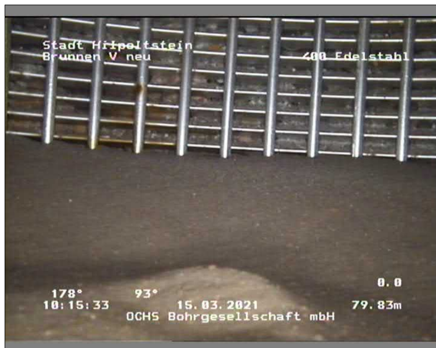
Foto: 101829_A.JPG, 00:16:48 79,83m, OK Boden
