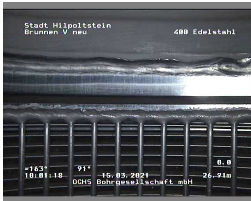
Foto: 100414_A.JPG, 00:03:30 26,91m, OK Filterrohr
