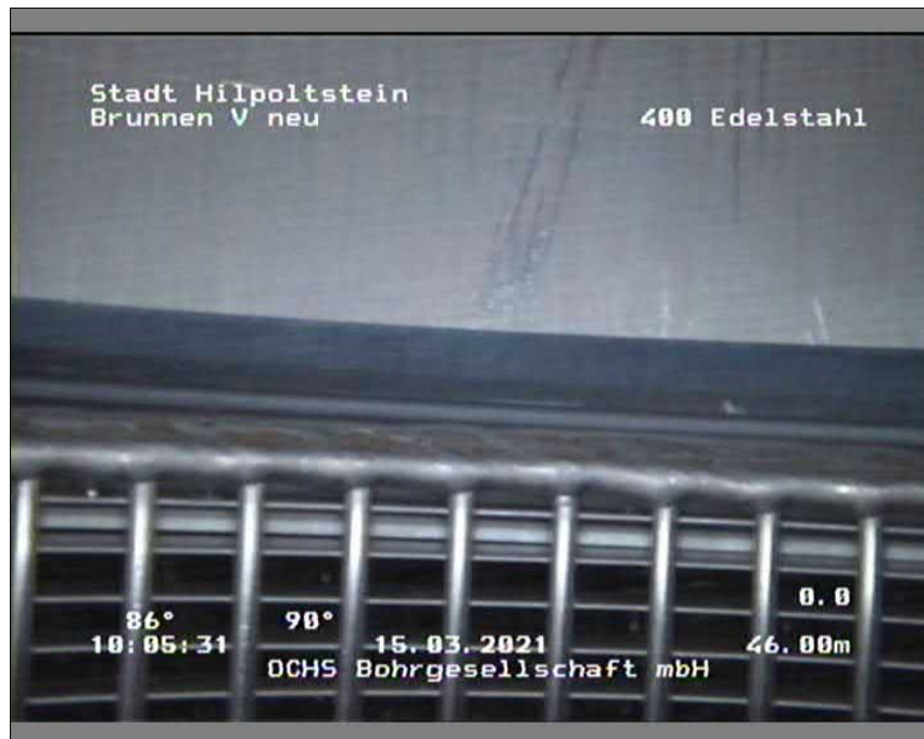
Foto: 100827_A.JPG, 00:07:24 46m, OK Filterrohr
